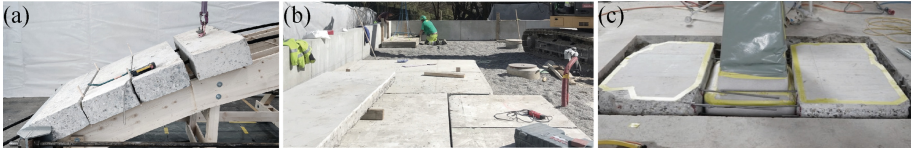
Fig. 2. RC reuse project built in Switzerland: (a) Re:Crete footbridge in Wallis, (b) carriageable pavement in Meyrin, and (c) column foundations in Zurich. Image credits: (a) EPFL; (b) FAZ Architectes; (c) baubüro in situ.
