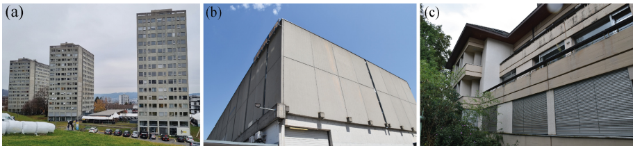
Fig. 5. Building case studies: (a) Zurich Triemli Stadtpital Personalhauser, (b) Basel Lagerhalle Erlenmatt Ost, (c) Basel Socinstrasse 59
