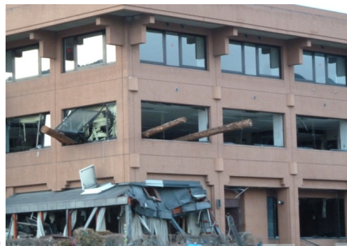
Figure 1. (a) Example of tsunami-structure interaction during the Indian Ocean tsunami (2004) [MThompson]; (b) Example of porous structure: Port building in Ofunato Chock et al. (2013) [Robertson].
