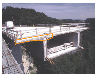
a) Bridge girder with cantilever
