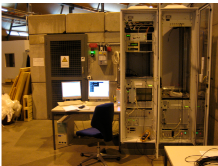
Figure 4.10: The test stand control system. Two 19" racks hold the controls hardware. The two VME crates can be seen in the bottom halves of the racks. The right rack is reserved for diagnostic controls hardware, the left rack holds network hardware, power supplies and vacuum controls.
