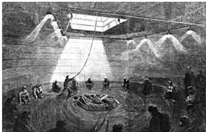
Figure 1. Loading the transatlantic cable into the ‘Great Eastern’ in 1865
