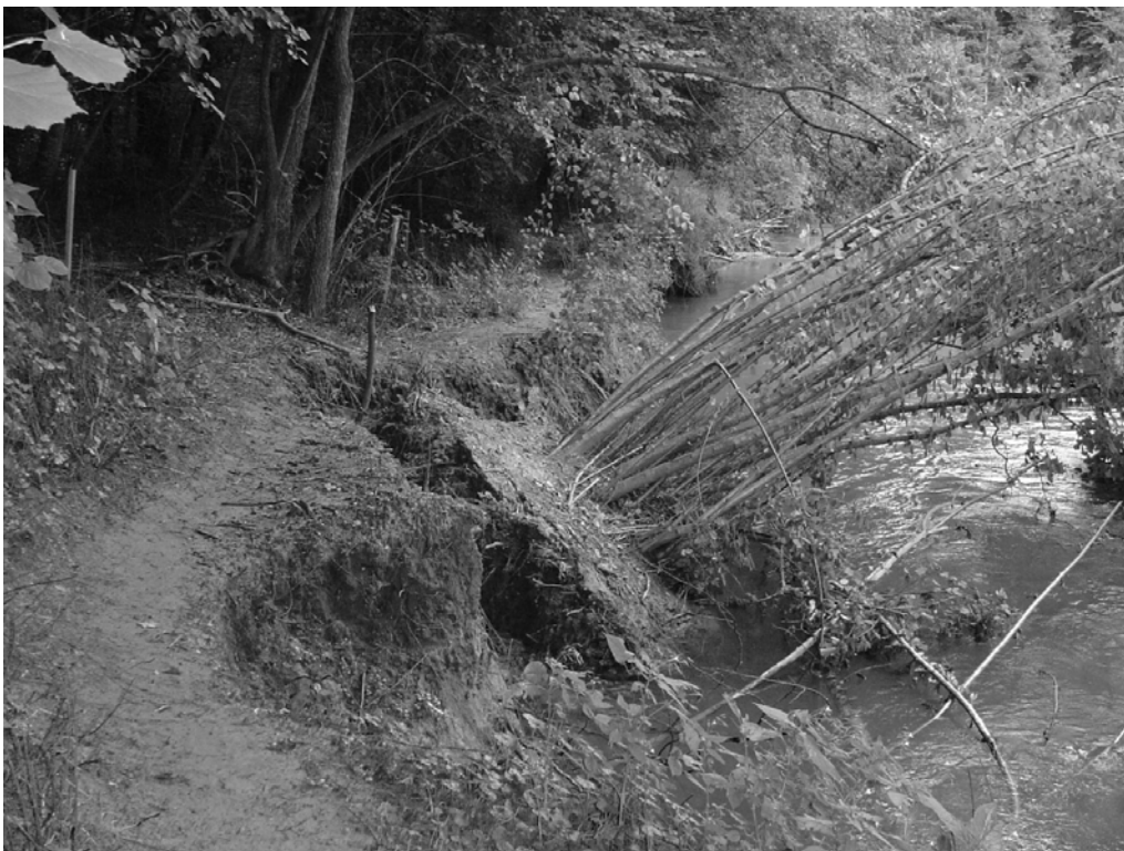
Figure 4.15. Tree cantilever failure of bend 7.2
