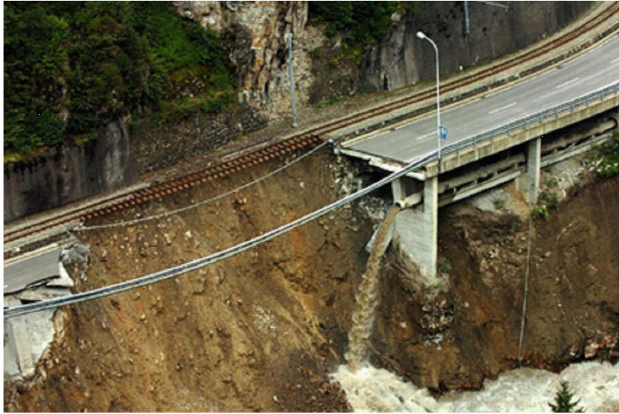
Figure 1.1. Destruction of the roadway leading to the mountain resort in Engelberg, Switzerland. The village was accessible only by helicopter during a two week period. (from Blick, 2005)
