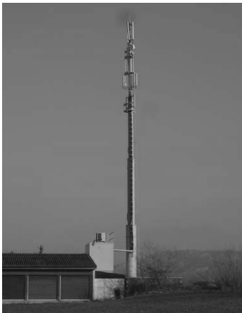
Fig. 3.4a: Example of a GSM BTS (macro cell) in an urban area (near Winterthur (CH)).
