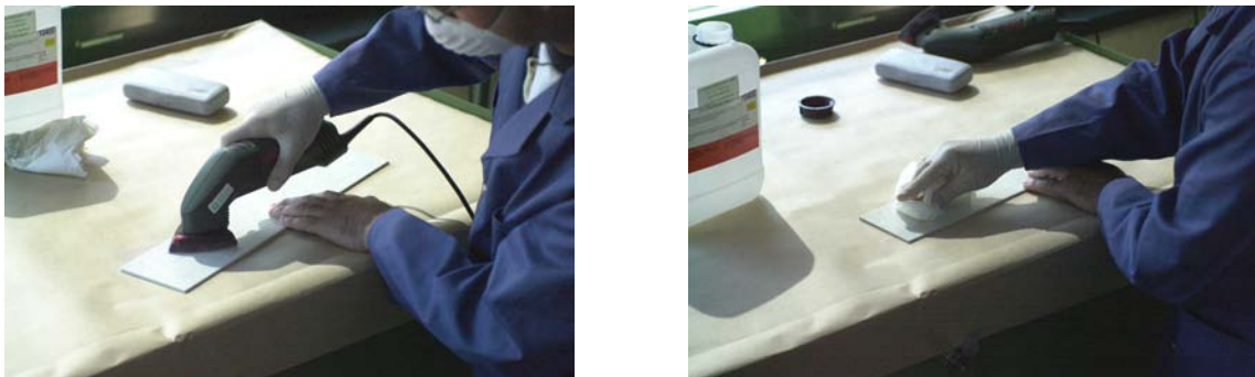
Figure 10 Surface treatment: (a) sanding, (b) degreasing
