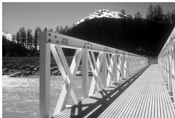
Figure 2.14: Redundant system – structural redundancy: Pontresina bridge (CCLab)
