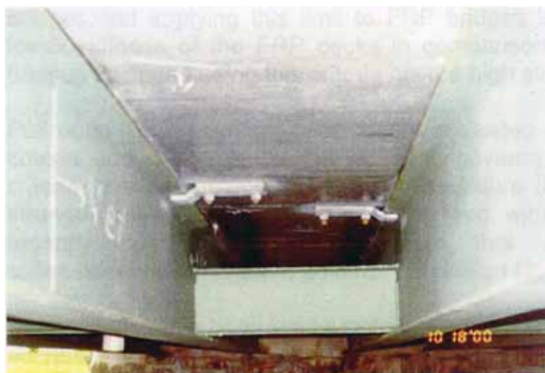
Figure 2.20: Hardcore deck clamped to the steel girder ; bridge over Mill Creek
