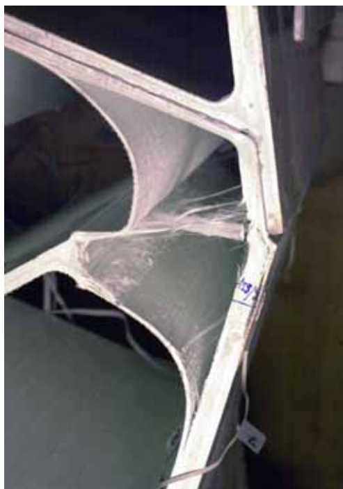
Figure 3.44: Detail of failure, specimen AS3
