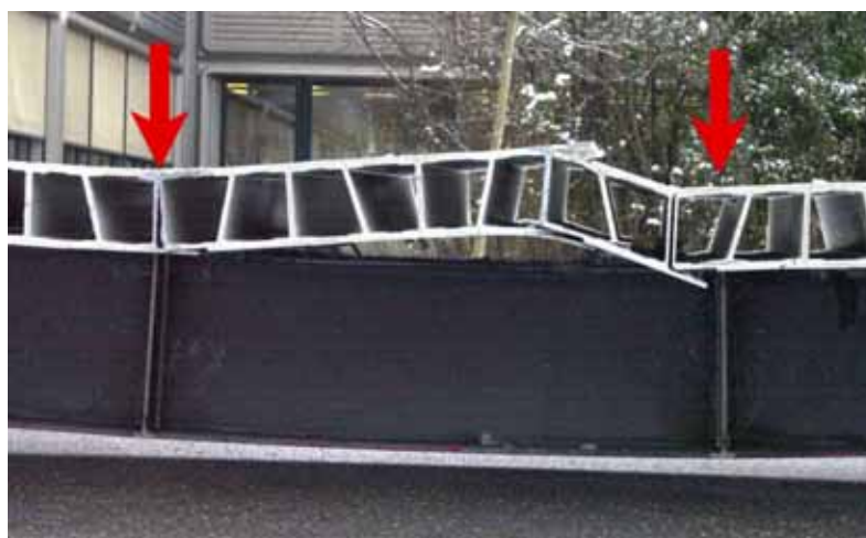
Figure 4.56: Secondary failure of girder Fix 2: buckling of the deck between jacks (residual deformation after demounting).
