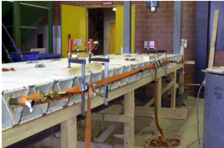
Figure 4.11: Clamped FRP elements of experimental girder Fix 3
