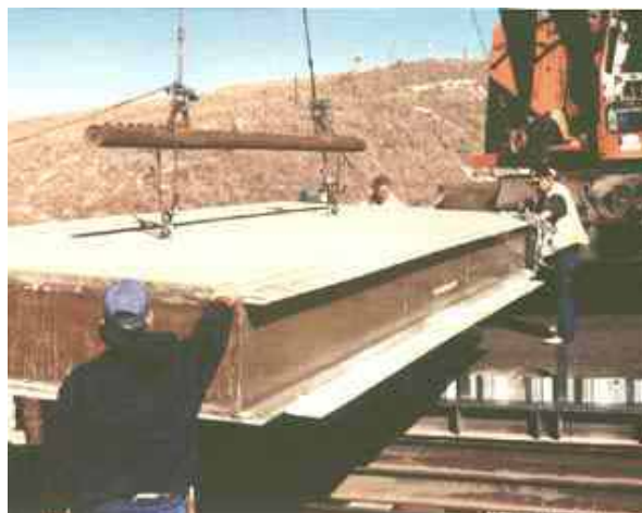
Figure 2.13: Installation of bridge deck over No-Name Creek
