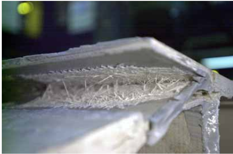
Figure E.31: Failure in the upper face sheet of an epoxy joint (near axis J - J) showing good adhesion but locations with no adhesive
