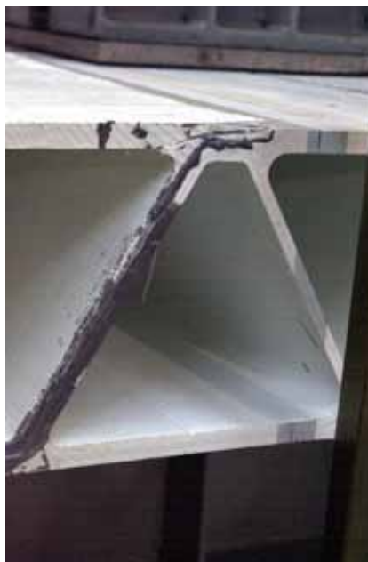
Figure 4.31: First failure of girder Fix 4 in a stepped joint of the upper face panel.
