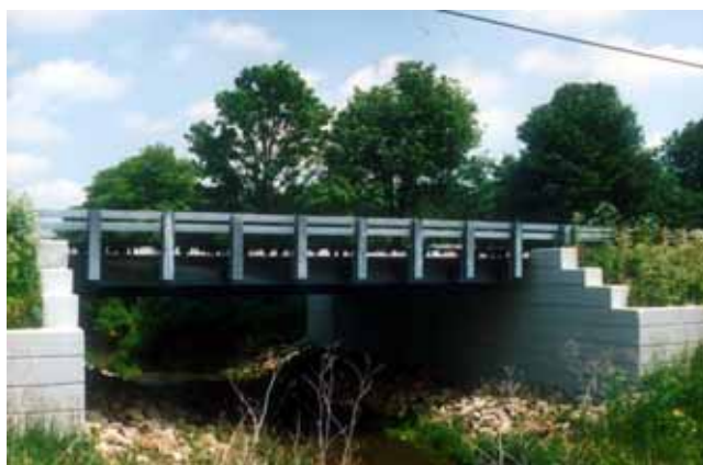
Figure 2.7: Bridge over Woodington Run (1999), Darke County
