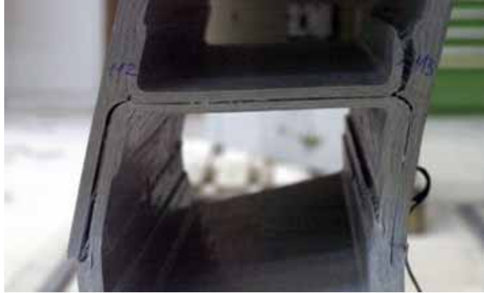
Figure 3.22: Delamination of web and failure of joint (Specimen 3cs).
