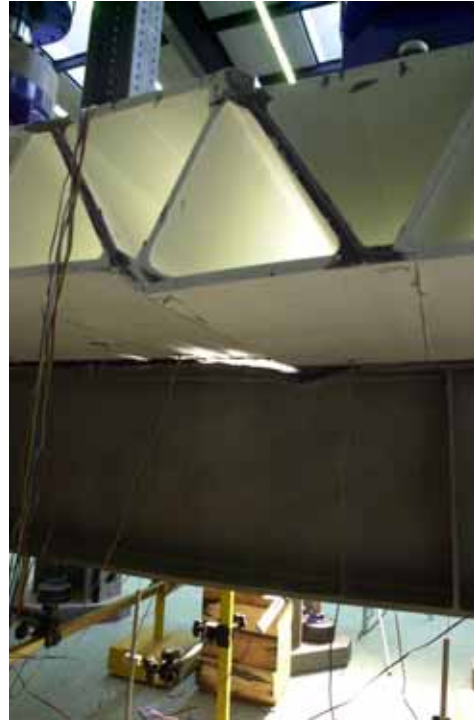
Figure E.13: Delamination of the bridge deck from the steel girder, Axis K - K
