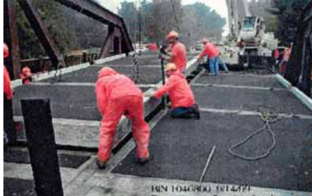
Figure 2.14: Installation of Hardcore bridge deck at Bentley's Creek
