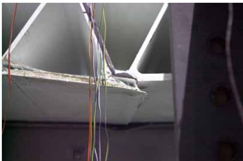
Figure E.19: Front view axis H - H with buckling of top steel flange
