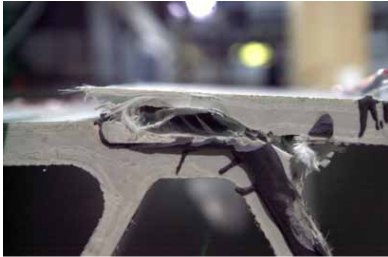
Figure E.17: Detail failure of upper face panel, axis H - H, front view
