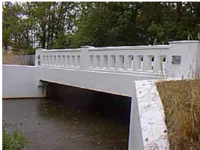
Figure 2.15: Completed bridge over Muddy Run
