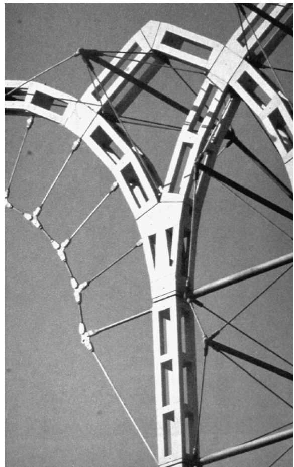
Fig. 24: Prestressed stone arch of the Pavilion of the Future, Seville. David Mackay and Peter Rice, 1992. (Rice)
