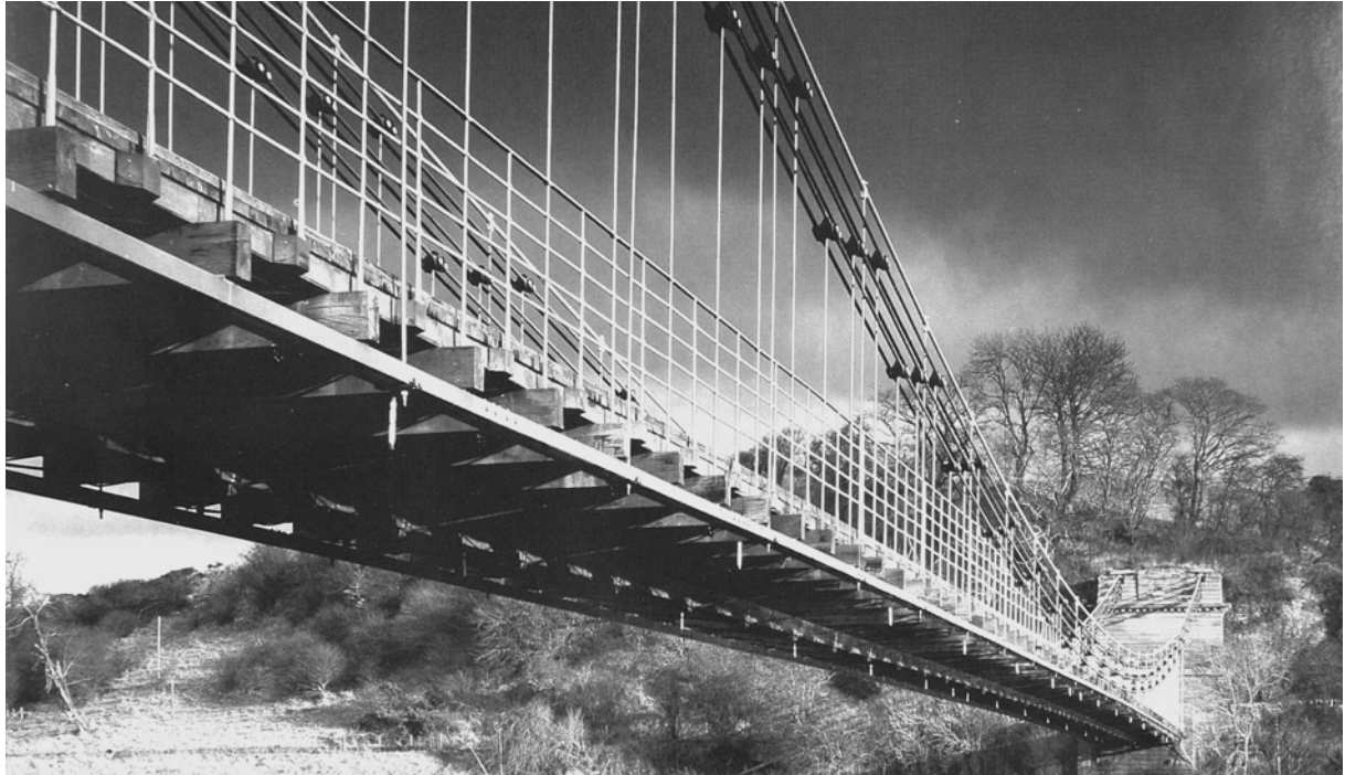
Fig. 13: Union Bridge, Samuel Brown, 1818. (Brown)
