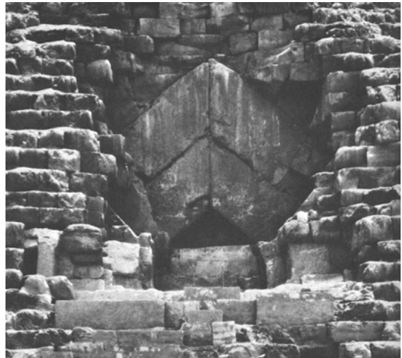
Fig. 6: Simple arch of two stones leaning against one another, north entrance to the Pyramid of Cheops, Giza. (Mainstone)
