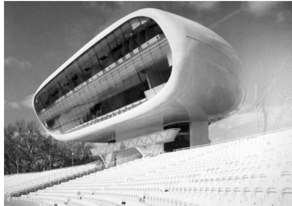
Fig. 41: The Media Center at Lord's Cricket Ground, London, 1998. Future Systems and Büro Happold. Semi-monocoque structure. (Future Systems)
