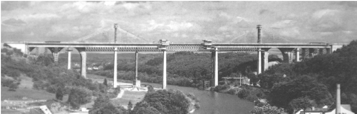
Fig. 45: Example of cantilever construction method using auxiliary cable stays. Image shows construction of the Lahntal Bridge at Limburg, Germany. The bridge was commenced at both abutments and advanced toward the center. (Wittfoht)
