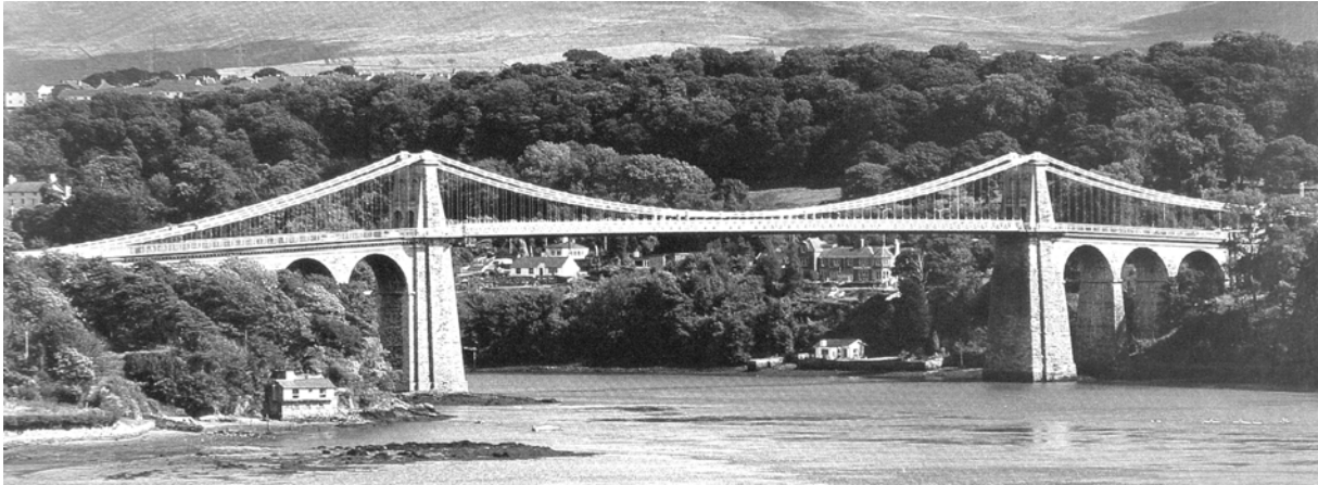
Fig. 31: The Menai Suspension Bridge. Completed 1826, Telford. (Brown)
