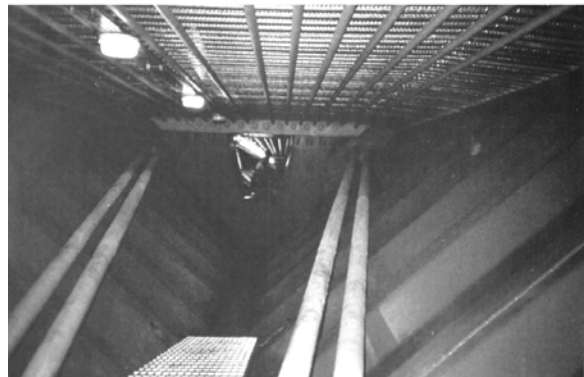
Fig. 71: Triangular section with closed webs of corrugated steel. Vallon de Maupré Viaduct at Charolles. (a) General view. (b) Inside triangular box girder. (SETRA)
