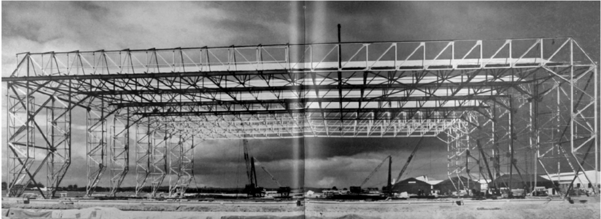
Fig. 39: De Havilland Avion Hanger, trussed aluminum frame structure spanning 61 m. James M. Monro & Son, 1955. (Peter)
