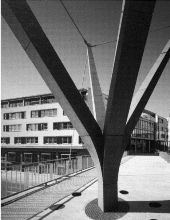
Fig. 25: Stone mast of a cable supported pedestrian bridge in Bad Homburg, Germany. Schlaich Bergemann & Partner, 2002. (Russell)
