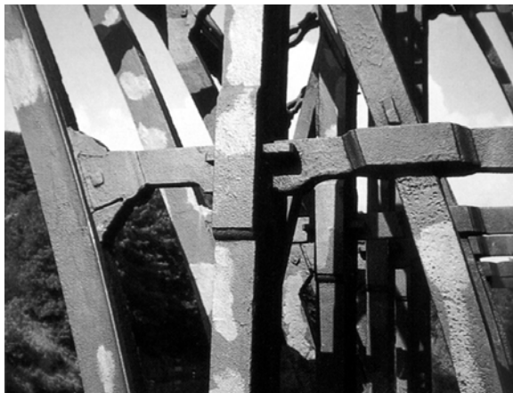
Fig. 43: Detail of Ironbridge showing timber-like connection. (Brown)
