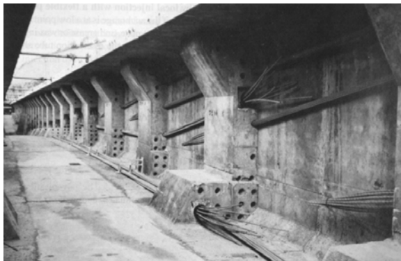
Fig. 74: Viaduct of Sermeaz, showing vertical arrangement of cables similar to geometry of Long Key Bridge without the same extreme eccentricities. (SETRA, after M. Virlogeux)
