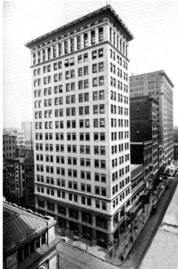
Fig. 16: Ingalls Building, 16 story reinforced concrete structure designed and built by the Ferro-Concrete Company, Cincinnati, 1902. (Collins)
