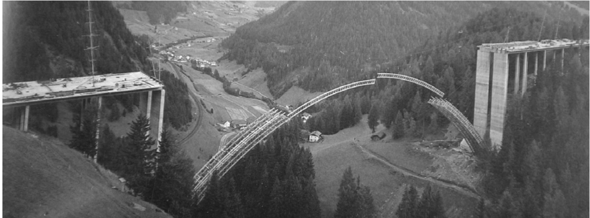
Fig. 38: Erection of the timber lattice truss centering with a 180 m span for the First Nösslach Bridge, Austria. (Wittfoht)
