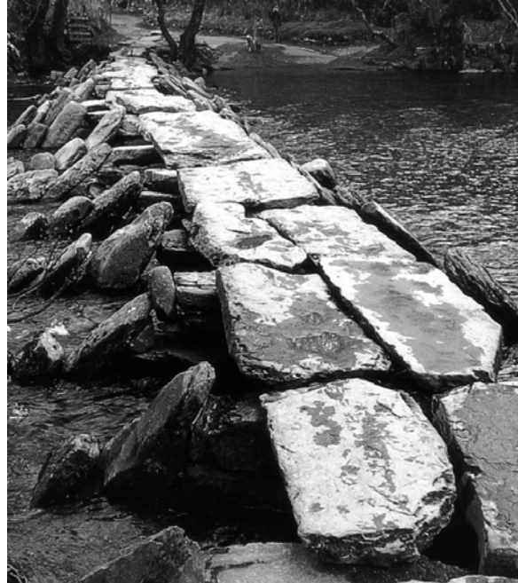
Fig. 26: Primitive bridge using flat stones that are simply supported. (Brown)
