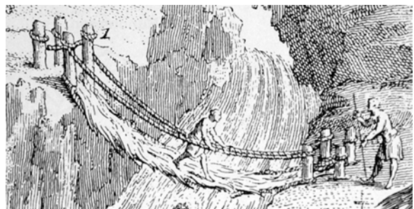
Fig. 3: Basic three-rope suspension bridge. (Brown)
