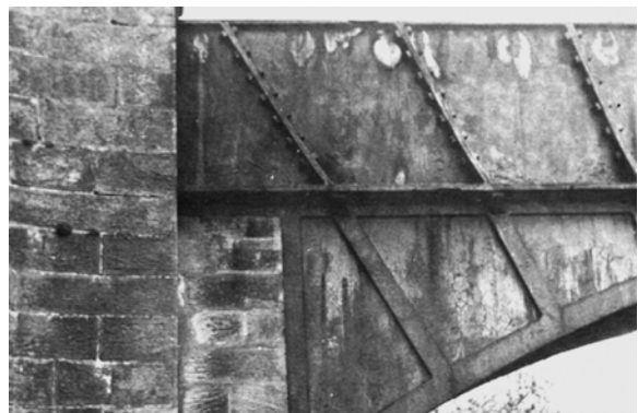
Fig. 21: Pont Cysyllte Viaduct, 1805. (Sealey)
