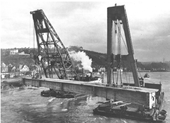
Fig. 39: 150 metric ton precast, Prestressed concrete girder being floated into position by enormous cranes for the bridge over the Rhine at Vallendar, Germany, 1959. (Wittfoht)
