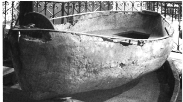
Fig. 4: Ferro-cement boat, Lambot, 1848. (Prade)
