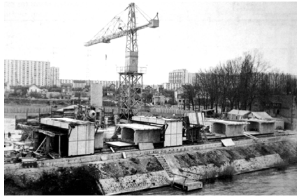
Fig. 56: Match-cast box girder segments in precasting yard for the construction of the Choisy-le-Roi Bridge, France. (Podolny and Muller)
