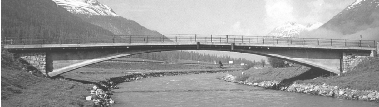
Fig. 36: Zuoz Bridge, first reinforced concrete box section bridge with plain spandrels, Robert Maillart, 1901. (Brown)
