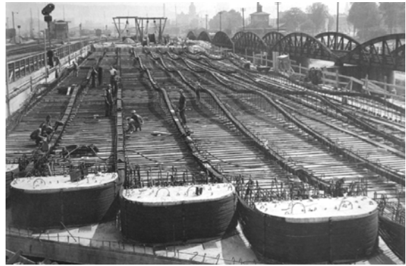
Fig. 34: Baur-Leonhardt prestressing system used in the first post-tensioned prestressed concrete railway bridge over the Neckar at Heilbronn, Germany, 1951. (Wittfoht)
