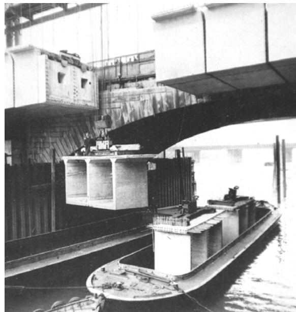
Fig. 52: New London Bridge being assembled using precast box-section segments. (Wittfoht)
