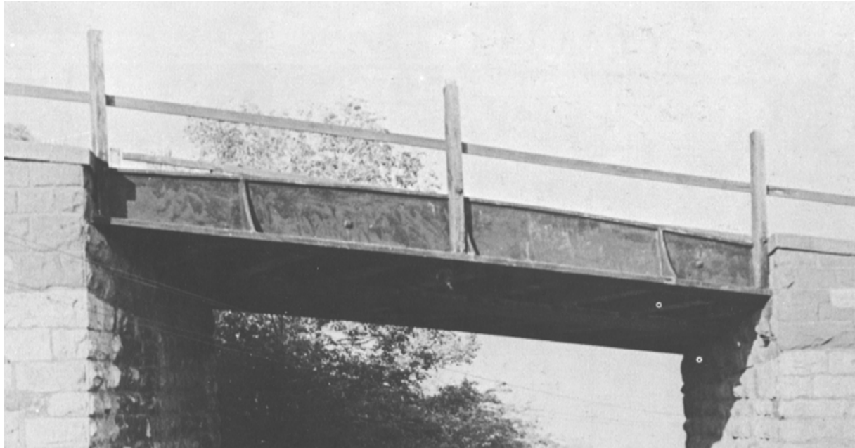
Fig. 32: Typical cast-iron girder bridge for railroads in England, early 19 th century. (Sealy)
