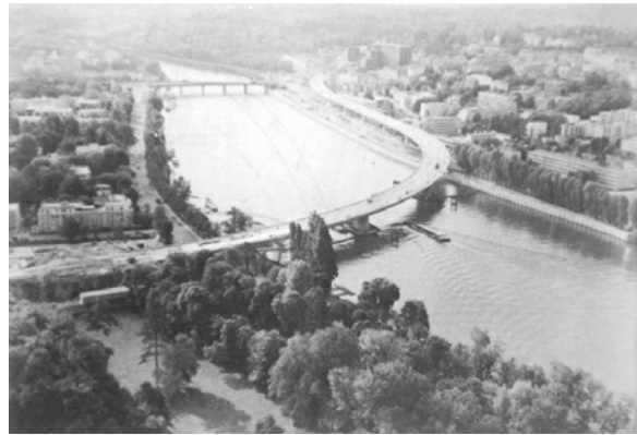
Fig. 60: Saint Cloud Bridge, on Paris Ring Road over the Seine River, France, 1975. General view showing difficult geometry and the use of three-dimensional pre-stressing to counter torsion. (Podolny and Muller)
