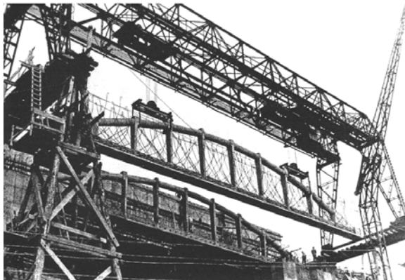
Fig. 24: Prestressed concrete roof girder with 30 m spans used to construct German submarine pen, 1943. (a) Cross-section of submarine pen. (b) Roof girder being lifted into place during construction. (Grote and Marrey)
