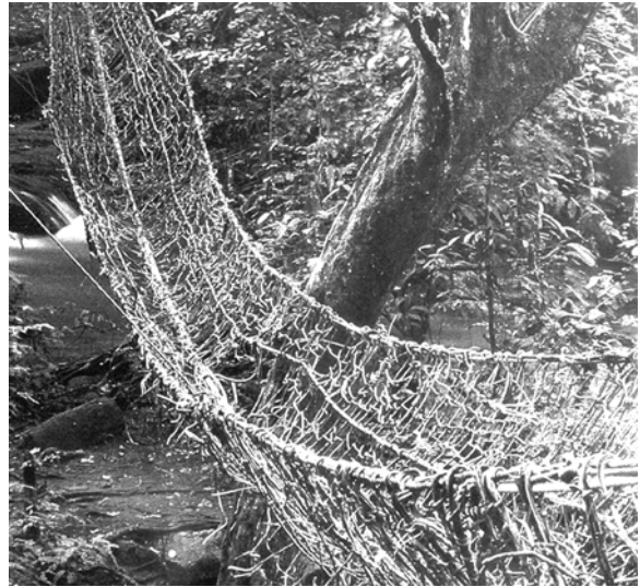
Fig. 1: Three-cable suspension bridge manufactured using vines. (Brown)
