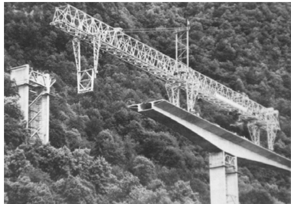
Fig. 61: Chillon Viaduct, Montreux, Switzerland. Construction view. 1970. (Wittfoht)
