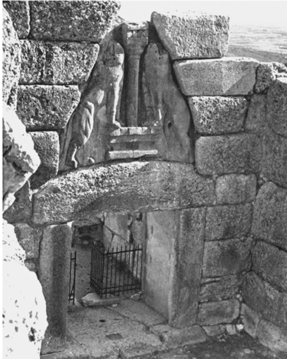
Fig. 15: Lion Gate, Mycenae, c.1300. The false arch relieves much of the load above the lintel. (Lawrence)
