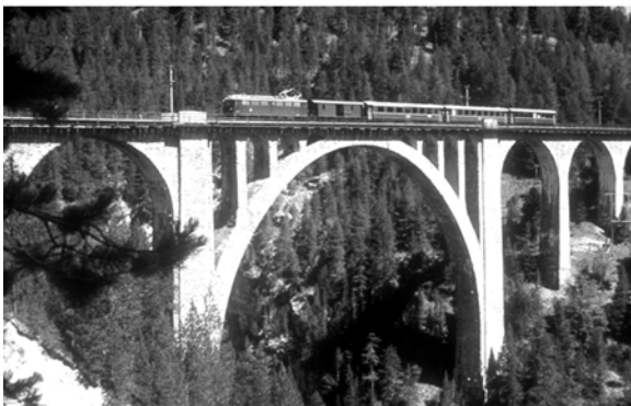
Fig. 23: Stone viaducts built at the turn of the twentieth century. Langwasser Viaduct (1902) and the Wiesener Viaduct (1908). These are among the slenderest constructions of their type. Both are located in Graubünden, Switzerland.
