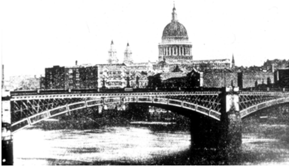
Fig. 5.13: Southwark Bridge, London. John Rennie, 1819. (Peters)
