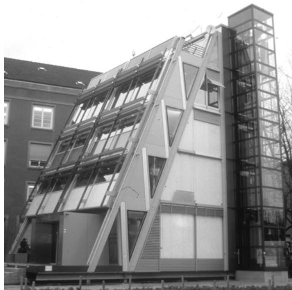
Fig. 6.31: Eyecatcher, Basel. Tallest all-FRP building at 5 stories. Artevetro Architects and CCLab, 1999.
