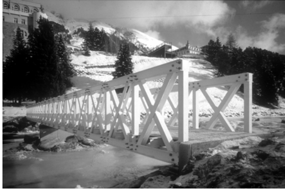
Fig. 6.22: All-FRP Pontresina Footbridge, Switzerland. CCLab, 1997. (CCLab)
