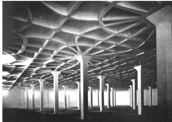
Fig. 5.7: Underside of floor slab of the Gatti wool factory showing isostatic stress lines, Rome, Pier Luigi Nervi. 1951. (Nervi 2 )
