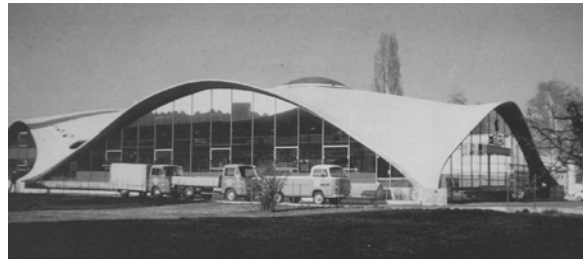
Fig. 4.25: Free-form, reinforced concrete thin shell. Sici Factory, Geneva. Heinz Isler, 1969. (Chilton)
