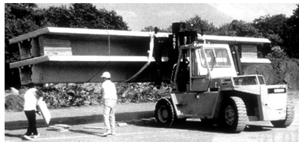
Fig. 6.20: All-FRP Smith Road Bridge, USA. Martin Marietta Materials, 1997. (CCLab, after Martin Marietta)
