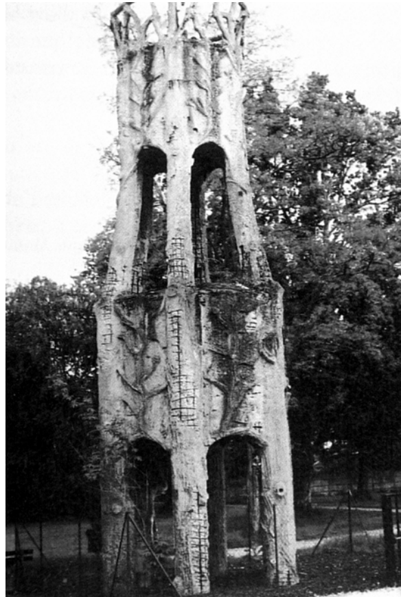
Fig. 5.10: Reinforced concrete water tower, Monier System. Joseph Monier, c.1876. (Bosc)
