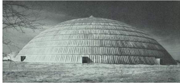
Fig. 4.26: Monocoque aluminum dome, diameter = 100 m. Meeting Hall, Longview, Texas. R.G. LeTourneau Co., 1953. (Peter)
