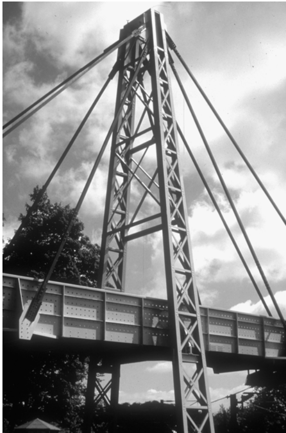
Fig. 6.23: Cable-stayed Fiberline Footbridge, Kolding, Denmark. Fiberline, 1997. (CCLab, after Fiberline)
