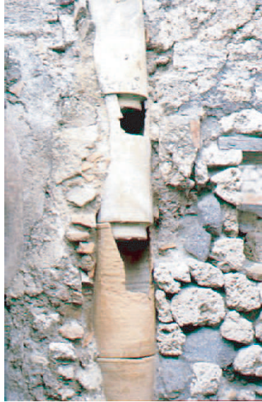
Figure 1.1: Clay heating ducts embedded in the wall of a house, Pompeii
