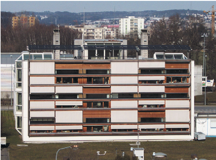
Figure 5.2: South facade view of the LESO experimental building
