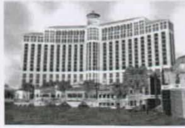
Figure II.III.23 The design group of Atlandia re-created the exterior and key interior areas of the hotel, which provided a realistic perspective of the project ( K. Moltenbrey, ref. [61]).
