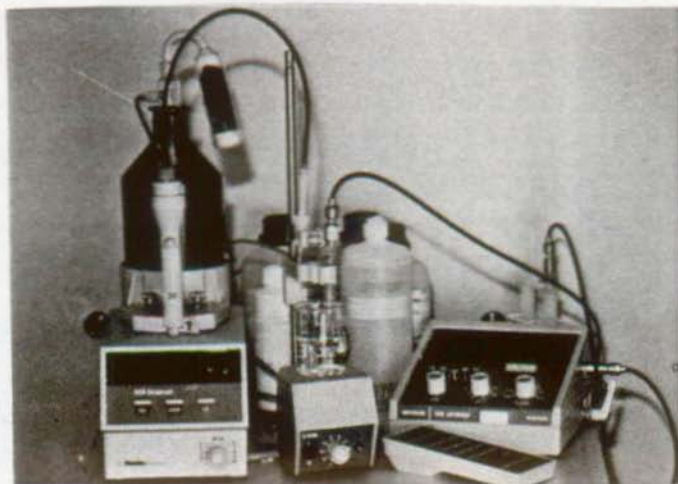
Figure 2.8 Experimental set for the titration of carbonate.
