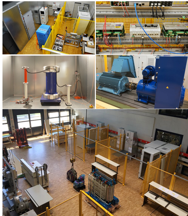
▲ Medium Voltage Power Electronics Laboratory
