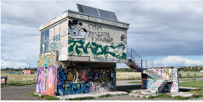
Figure 4. The “Plattenvereinigung” project reused precast panels and staircase elements from East-German and West-German buildings (2010). Credits: EPFL.
