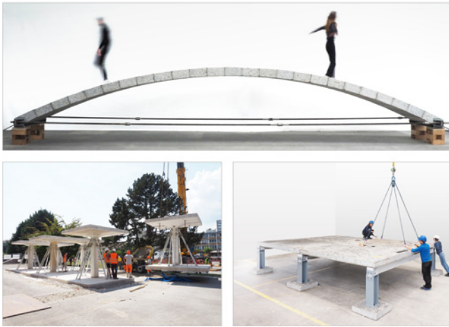
Figure 5. Geometry of reused pieces cut from cast-in-place concrete structures: blocks (top), assemblies (left), slab or wall elements (right). Credits: EPFL.
