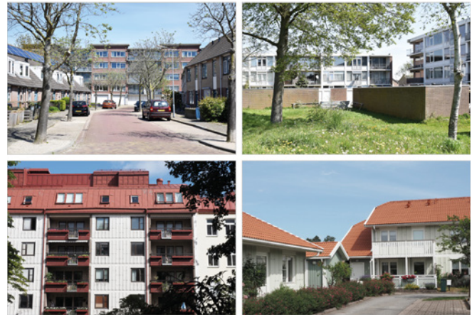
Figure 3. On the top left is the remaining donor building in Middelburg (NL), of which the upper-level panels were carefully dismantled and reused to build 3 mid-rise housing buildings in the same city in 1986, shown on the top right.
