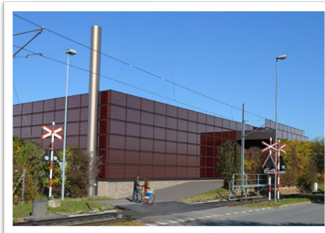
EPFL's new DC in the CCT building with PV generation, water cooling and heat recovery for heating of the campus
