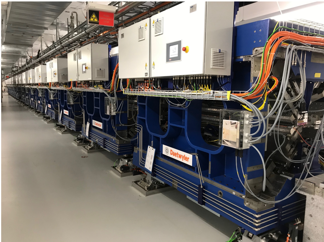
Figure 3.5: Athos undulator at SwissFEL. The Athos undulator is 44 m long, comprising 16 modules. Each module measures 2 m in length, with 0.75 m intersections between them [59].
