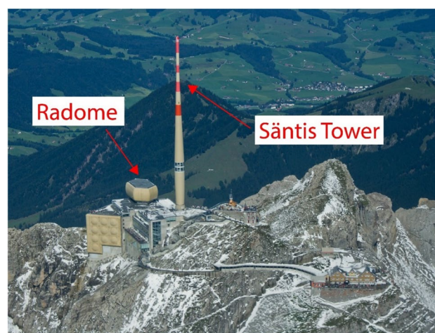
Figure 1. Photo of the Säntis peak, with arrows indicating the Radome, which houses the electric field probe and scintillators, and the Tower, where the current and current-derivative sensors are located. Image reproduced from Rachidi and Rubinstein 10 (Fig. 2) with permission.
