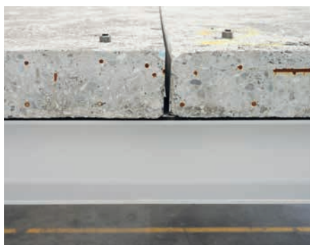
↑ FIGURE 8: FLO:RE building floor: connection detail between reinforced concrete slab elements and steel beams
