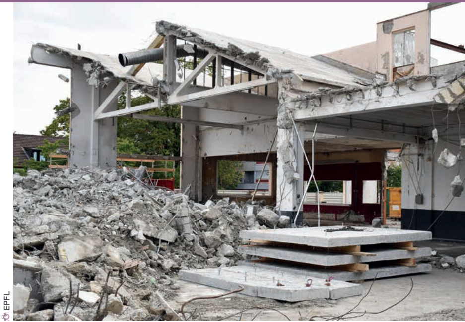
FIGURE 1: Concrete elements extracted by sawing before demolition of building, stored next to commonly produced concrete rubble
