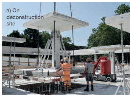
↘ FIGURE 11: rebuiLT pavilion: lifting of slab-column assemblies
