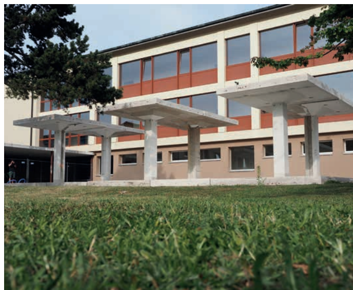
→ FIGURE 9: rebuiLT pavilion: reclaimed reinforced concrete elements in their final position
