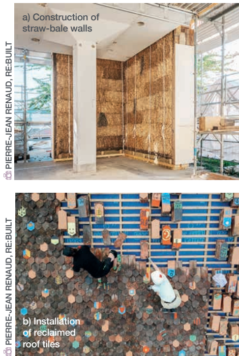
↑ FIGURE 12: rebuiLT pavilion: construction
