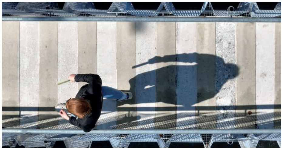
FIGURE 4: Re:Crete footbridge, with railings and waterproofing strips, used by pedestrian to cross a river in Switzerland
