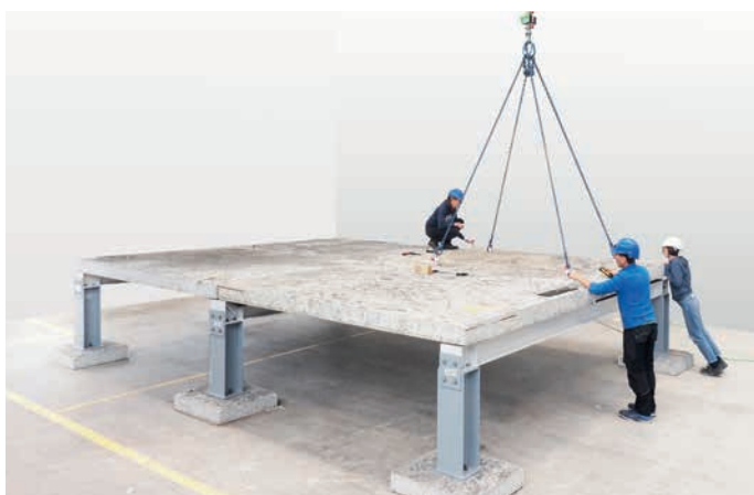
← FIGURE 6: FLO:RE building floor: extraction of concrete elements and steel beams
