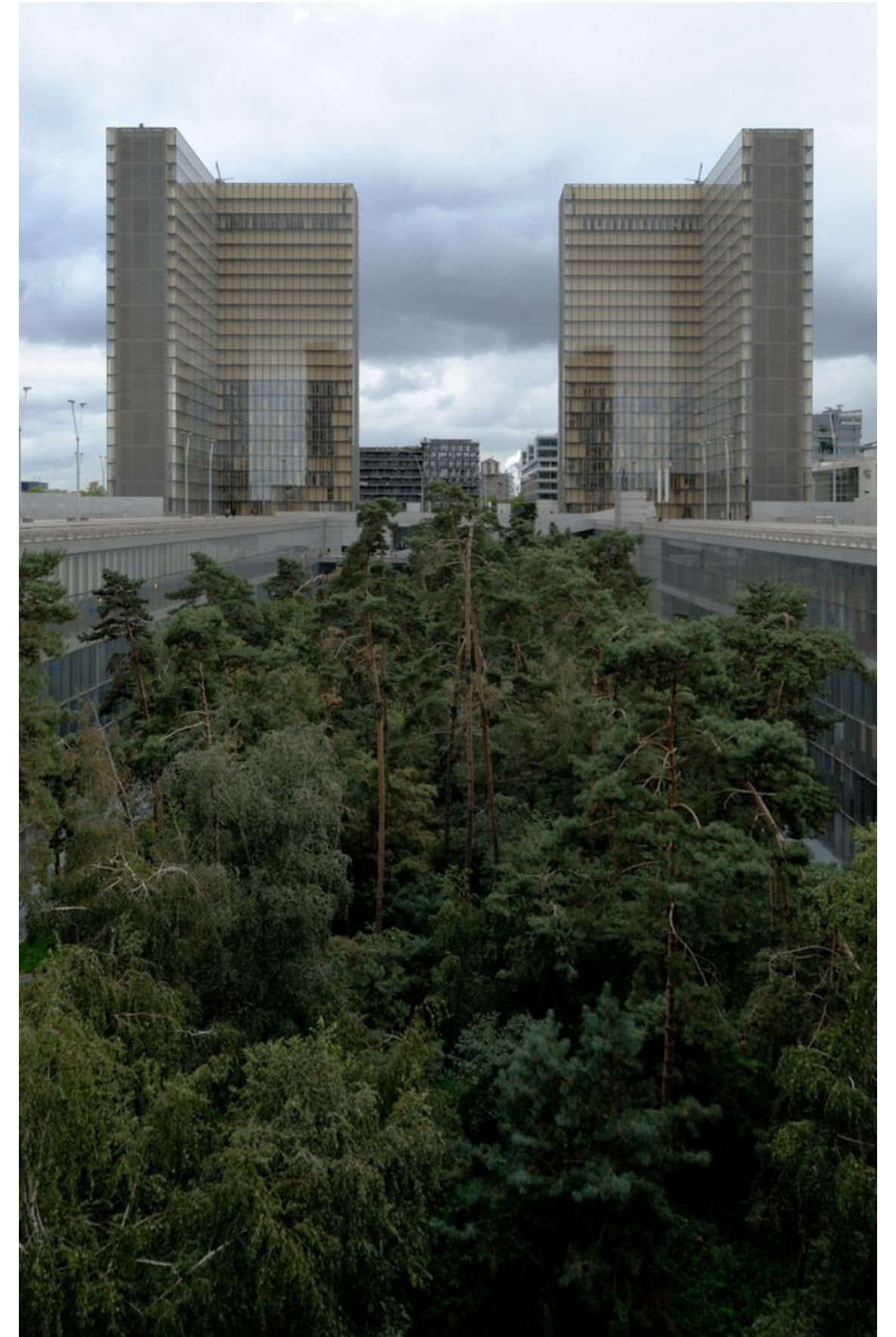
Figure 21: National Library of France (Archidailiy, 2011) 21
