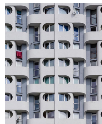
Façade of one of the buildings on the Manhattan housing estate
