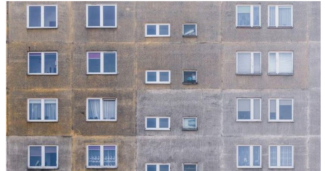
Façade of the WUF-T system building
