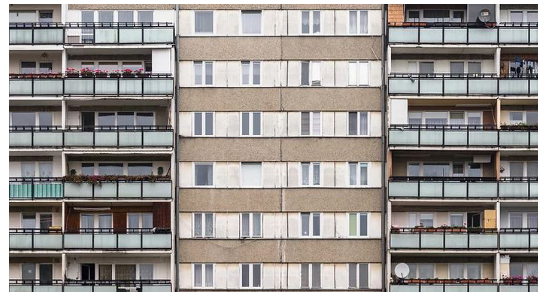
Façade of the OWT-67 system building
