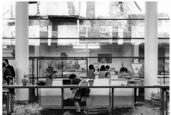
fig. 10 The workers working on the market.
