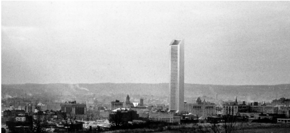
57. Kevin Roche, John Dinkeloo and Associates, Worcester County National Bank Tower, Projet initial, 1969
