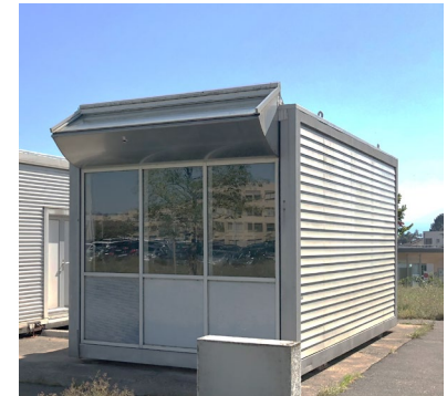
Test room from outside
