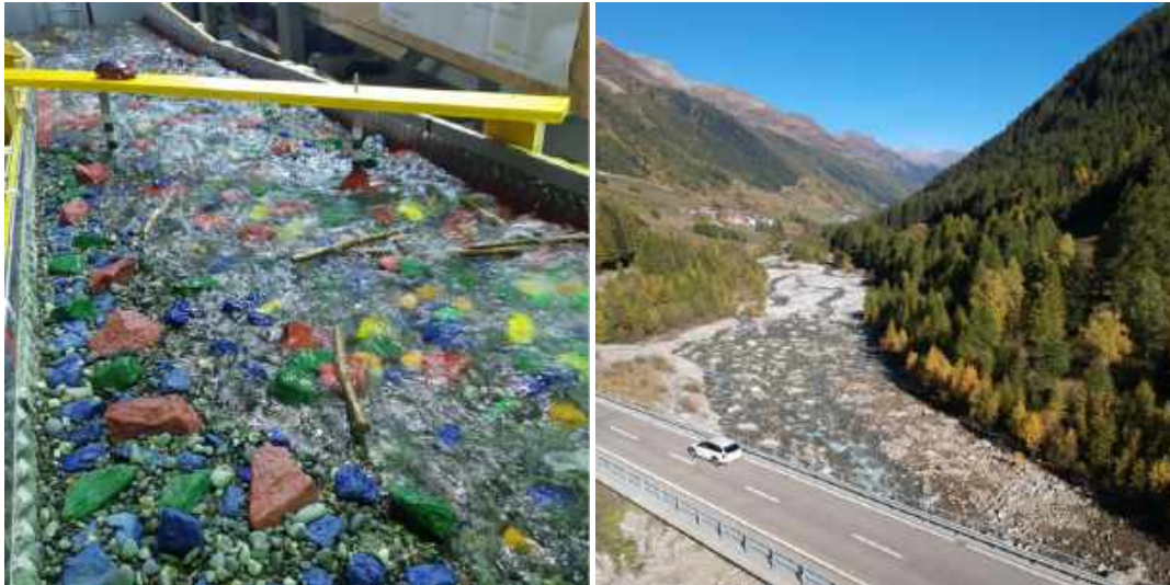
Figure 1.2: Dynamic ramp on the Ticino at Ronco Bedretto in the physical model at Laboratorio 3D (left) and after realization (right) (C. Tognacca et al., 2021).
