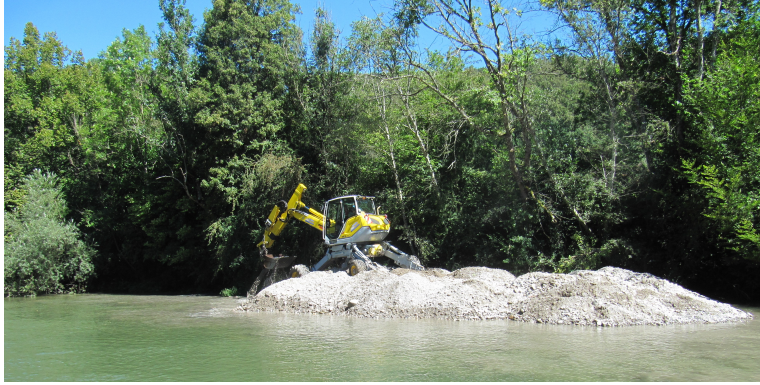
FIGURE 3.4 – Installation of sediment deposits in 2016.
