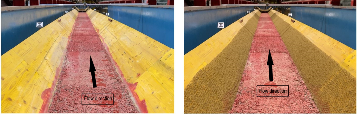
FIGURE 4.10 – Channel in its initial state (left) and after the installation of the geonet (right). Both pictures are taken in the run section, looking in the downstream direction. The black arrows show the flow direction.
