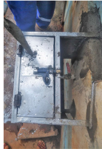
Figure 12: Cage for chlorinator, Mitamisyi.
