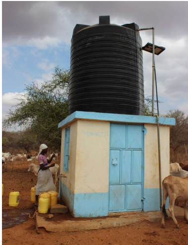
Figure 10: Water kiosk without chlorinator, Mitamisyi.
