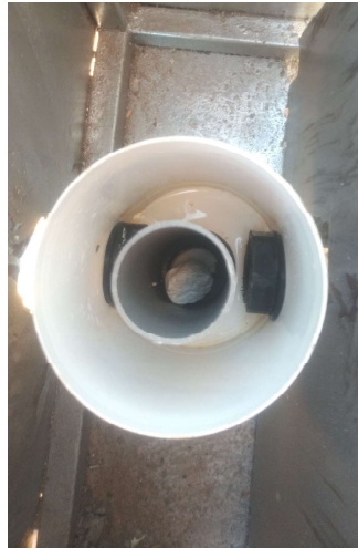
Figure 11: AkvoTur chlorinator, Mitamisyi.
