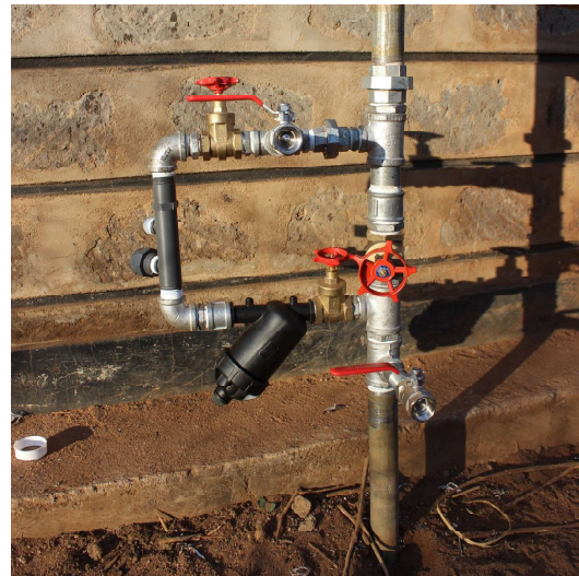
Figure 38: BlueTap bypass without the chlorine doser, Mumo.
