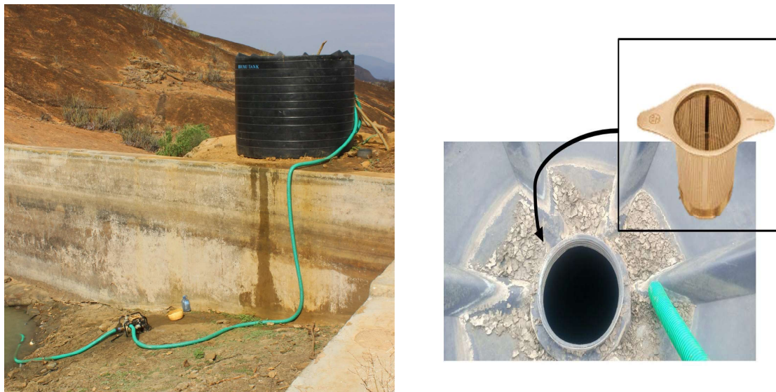
Left: tank of the Kyuso rock catchment and water pump powered by petrol. Right: upper part of the tank without lid, the water was pumped inside the tank using the green pipe; a picture of a filter is shown in the box.
