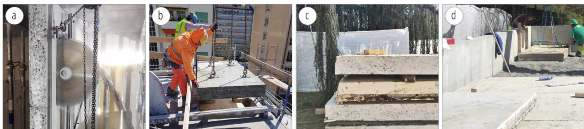
Figure 1 – Processes to reuse concrete: extraction (a, b), preparation and storage (c), installation (d). Credits: (a) EPFL/SXL; (b) Ingeni SA, (c,d) FAZ Architectes.
