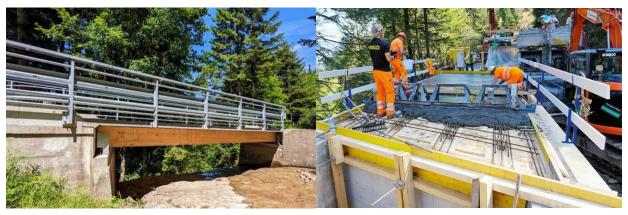
Figure 2 Presentation of the Fruttli Bridge and casting of the UHPFRC deck slab.
