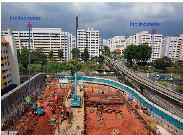
Fig. 6 Bukit Panjang hawker center excavation. Courtesy of Lian Soon Construction PTE LTD
