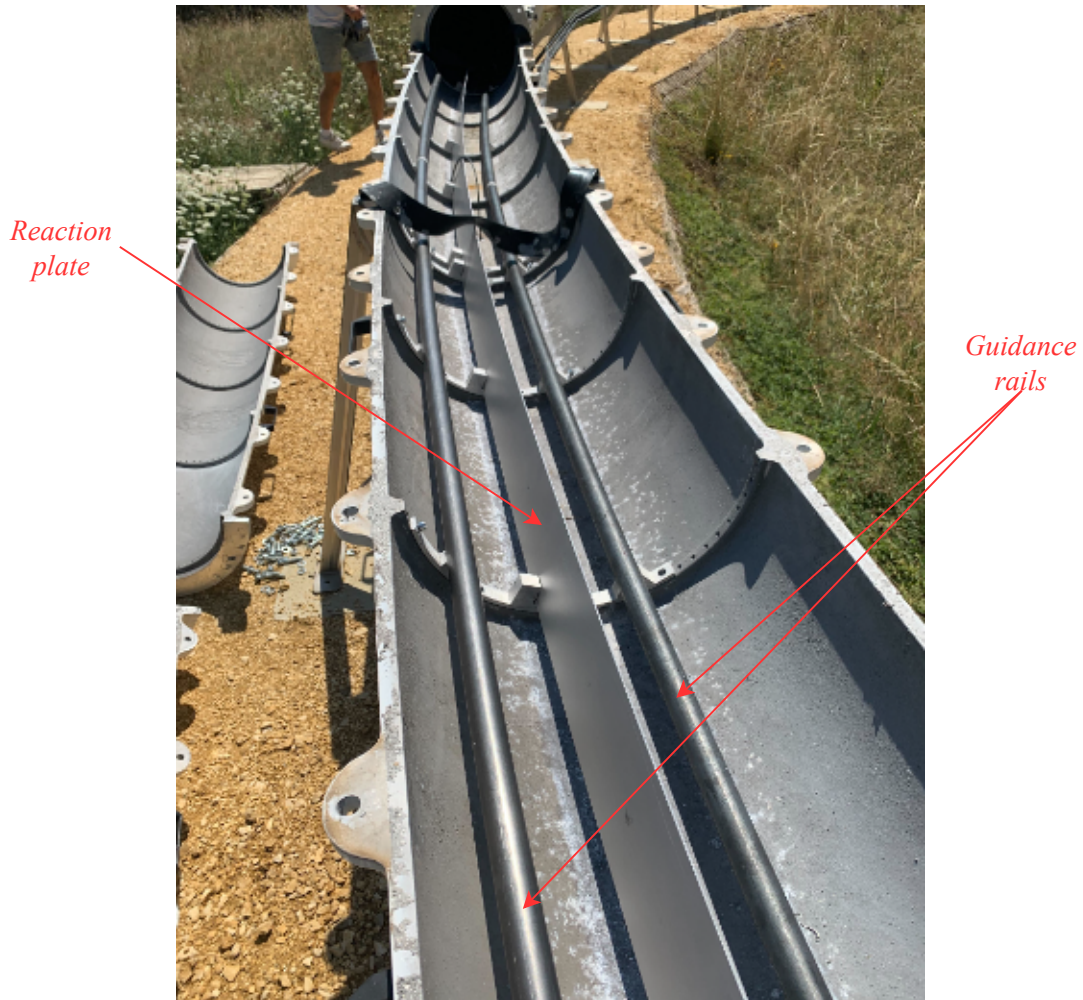
Figure 5.3: The rail design of the EPFL RS hyperloop test infrastructure.
