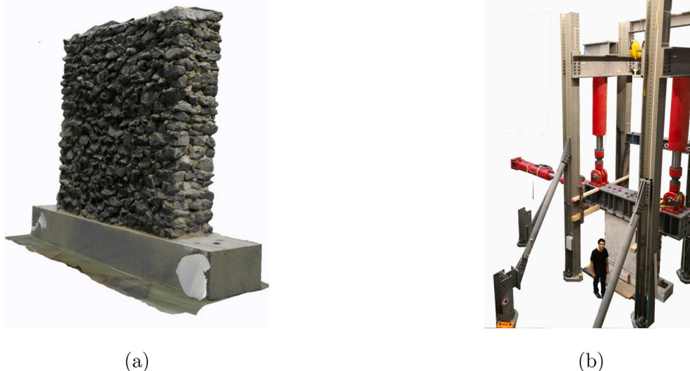
Fig. 3. Stone masonry walls: (a) Multi-leaf stone masonry wall built for laboratory testing and (b) corresponding test setup [15].
