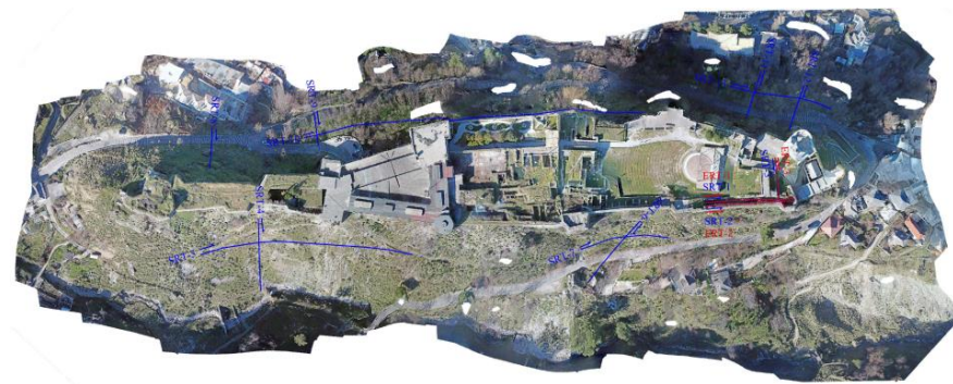
Figure 7. Location of seismic refraction (SRT, in blue) and electrical resistivity tomography (ERT, in red) profiles. (Photo credit: GEA, based on photo by Rand Eppich).
