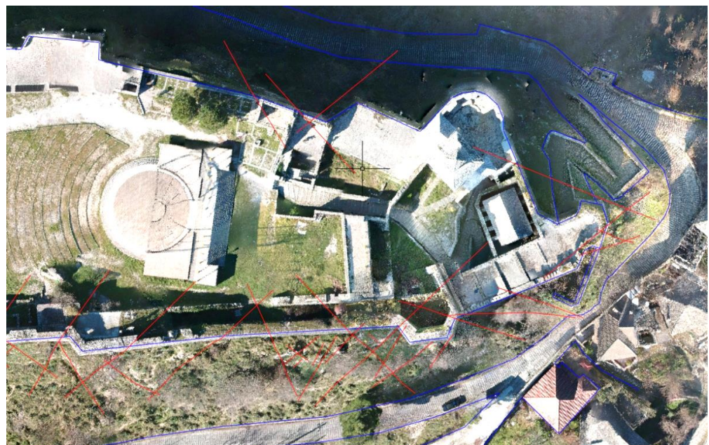
Figure 4. Detailed image of main joints in the conglomeratic around the tower located at the north-eastern end of the fortress (in red). Blue lines mark the outline of the fortress and the roads below. (Photo credit: GEA, based on photo by Rand Eppich).
