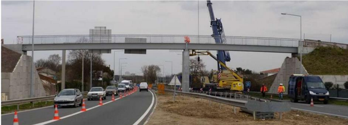
Figure 1. Pedestrian FRP Bridge, Saint-André de Cubzac, France, ©Photo P. Charbonneau.
