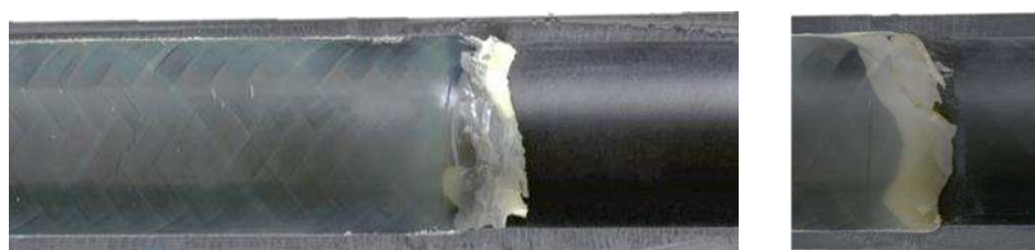
Figure 8. Liner Integration: End-plug area of BSP 5 (left); Liner delamination of BSP 4 (right)
