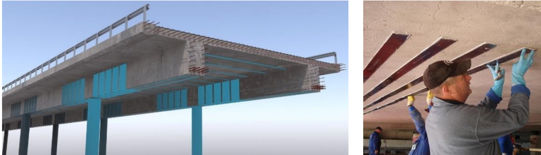
Figure 1. CFRP laminates and sheets strengthening of bridge and building structures [9].
