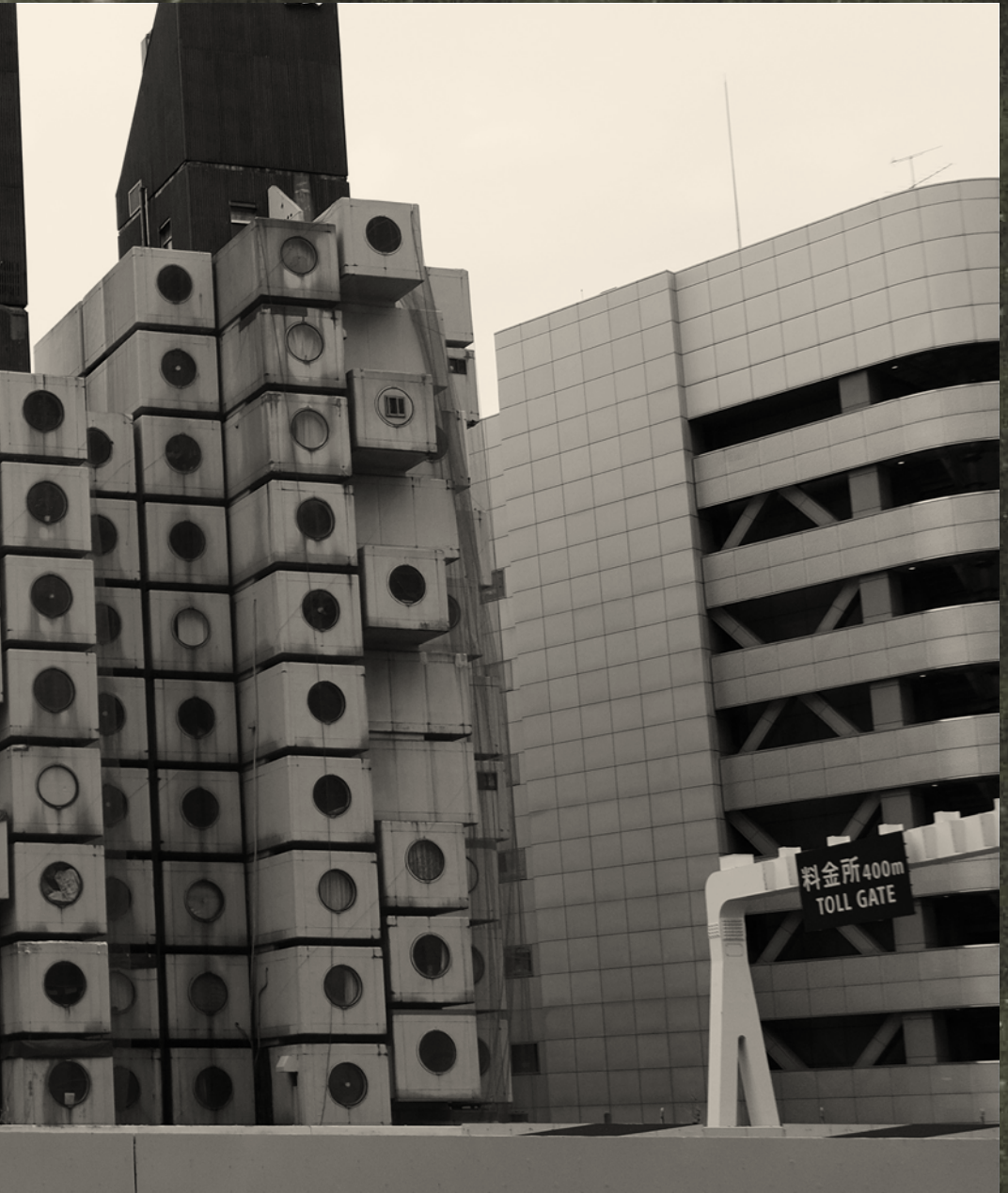
Nakagin Capsule Tower, view from outside in 2019. No Capsules have ever been replaced since its construction in 1972
