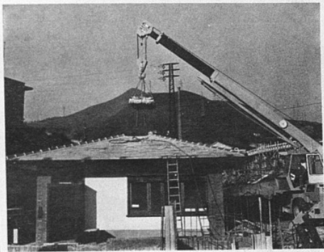
Atrium roof, Genova 1973
