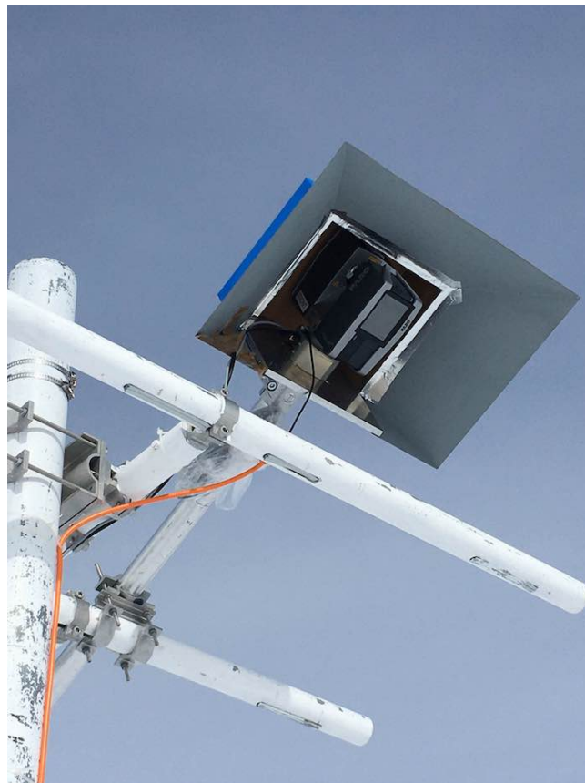
Figure A.6: The scanner set up seen from below
