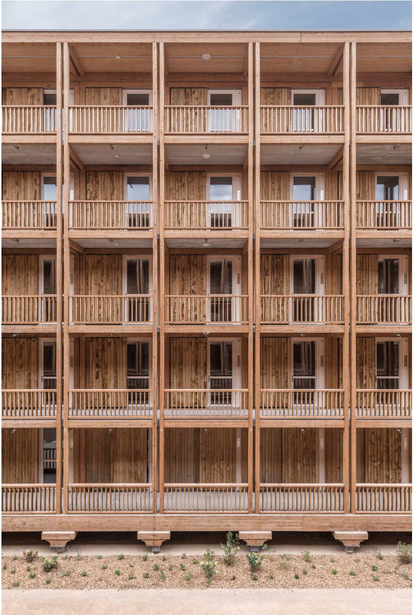
Foyer Rigot - façade © acau architecture sa fig. 28
