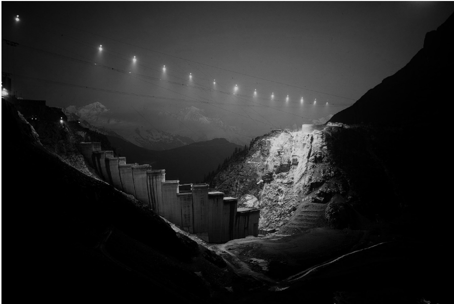
[Fig.5] Construction du barrage d'Eposson, 1971
