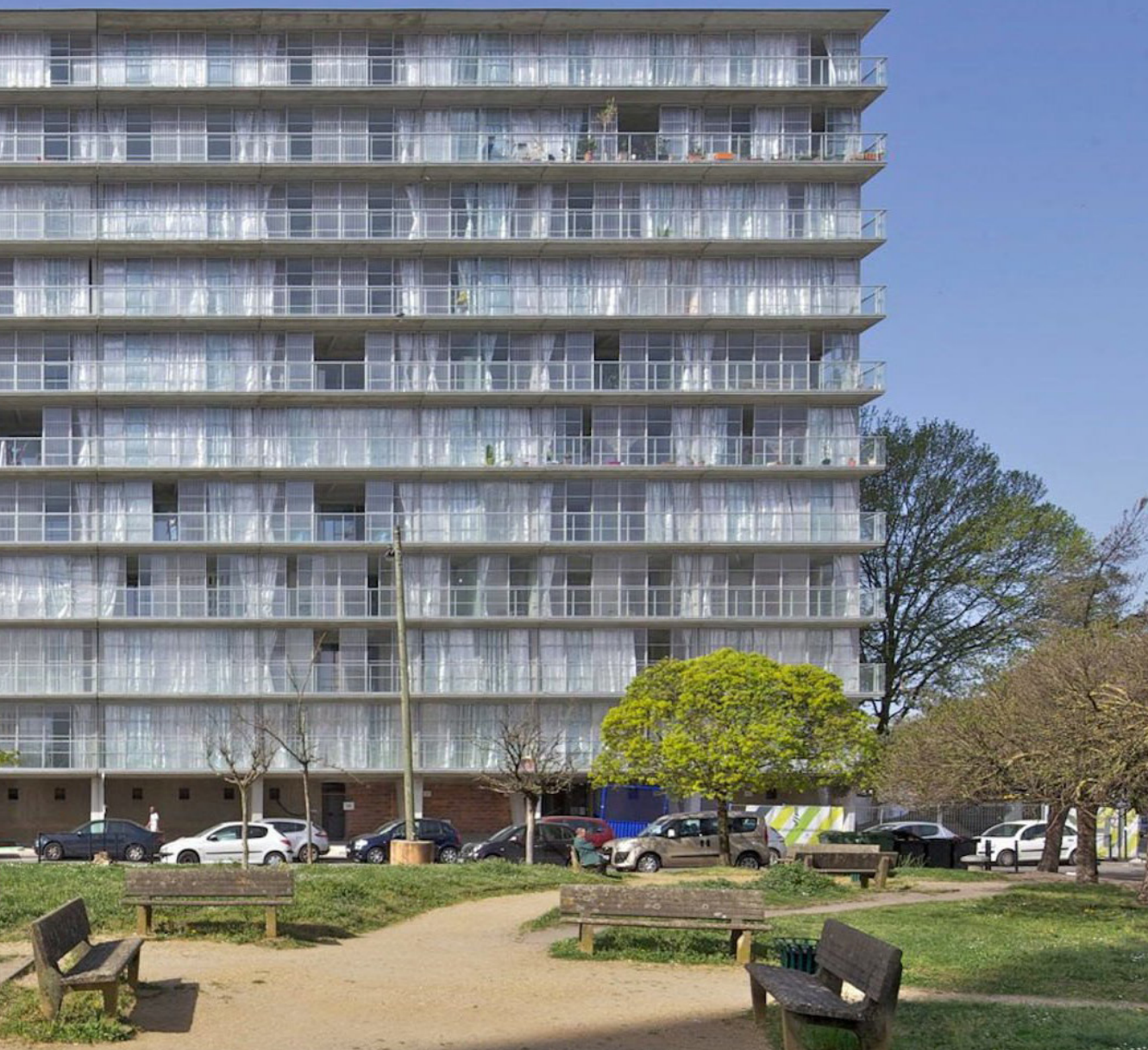
Philippe Ruault. The new, transparent south facade of one of the high-rise buildings that date from the 1960s. Photographie. Phillippe Ruault, Nantes. Baunetz_Knowledge. Avril 2015. [Consultée le 14 Janvier 2022]. https://www.baunetzwissen.de/bauphysik/objekte/wohnen/wohnhochhaeuser-cit-du-grand-pare-in-bordeaux-7214447
