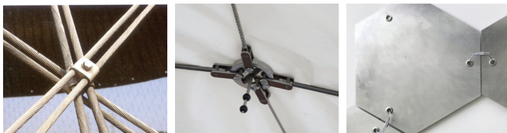
Figure 2: Left: Connection detail of the cooling tower of Schmehausen, see Schlaich and Bergermann (2004). Middle: connection detail of the Nest Hilo prototype, see Mendez Echenagucia et al. (2019). Right: Early prototype of connection detail of the Canopy Pavilion.
