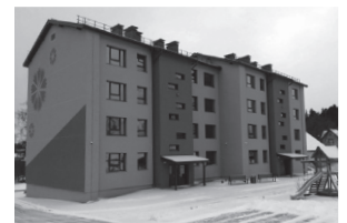
FIG 3.1 Apartment building renovation in Smiltene Source: Smiltenes NKUP
