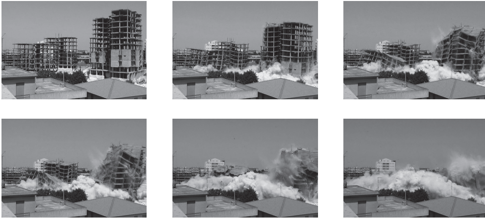
FIG 7.1 DEMOLITION#1 squatter, 2011 stills from a 3 min and 30 sec long video.
