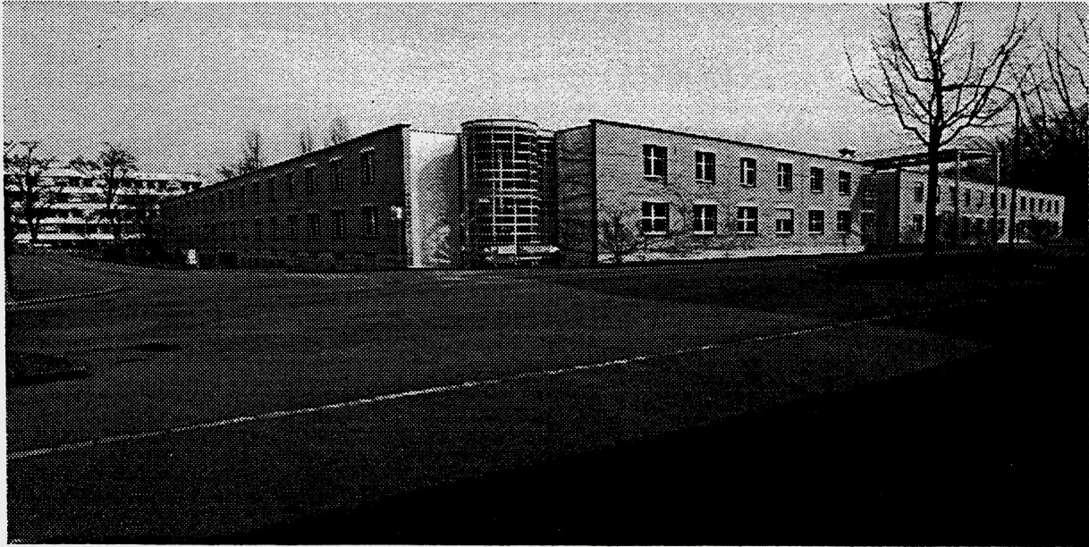
Figure 2.12: External view of the Reiterstrasse building (northwestern and southwestern facades)
