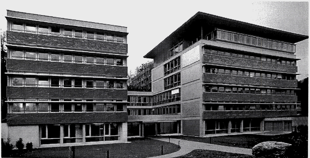
Figure 2.6: External view of the EOS Headquarters (southwestern facade)
