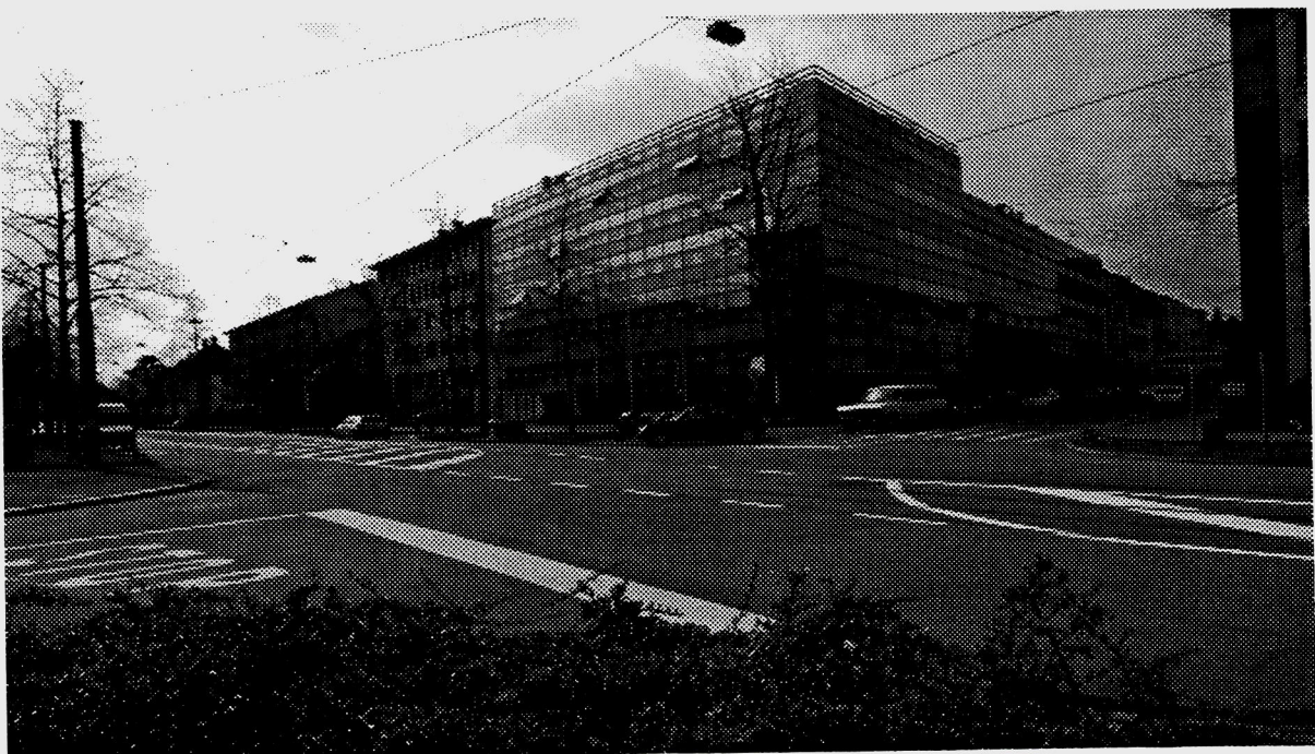
Figure 2.21: View of the CNA/SUVA building (northeastern facade)
