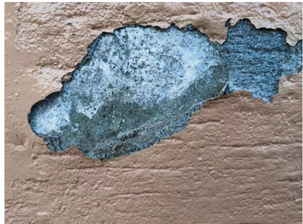
Fig. 2-6 Spalling damage examples caused by sodium sulfate crystallization: a) Surface scaled on a concrete foundation stem wall coated with latex paint [33], b) A building wall spalled with sodium sulfate deposit, coated with paint found in Pully, Switzerland.
