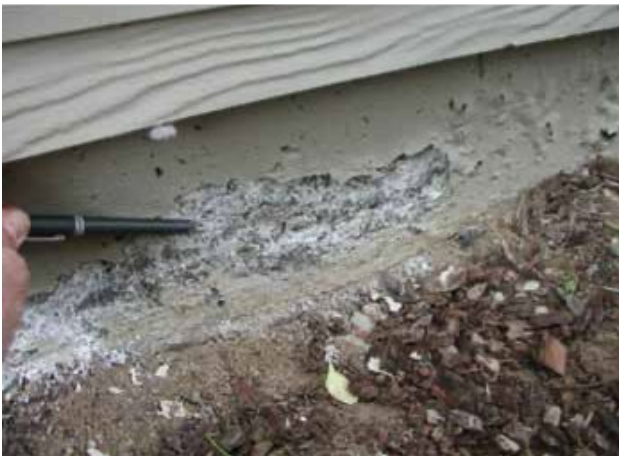
Fig. 2-6 Spalling damage examples caused by sodium sulfate crystallization: a) Surface scaled on a concrete foundation stem wall coated with latex paint [33], b) A building wall spalled with sodium sulfate deposit, coated with paint found in Pully, Switzerland.
