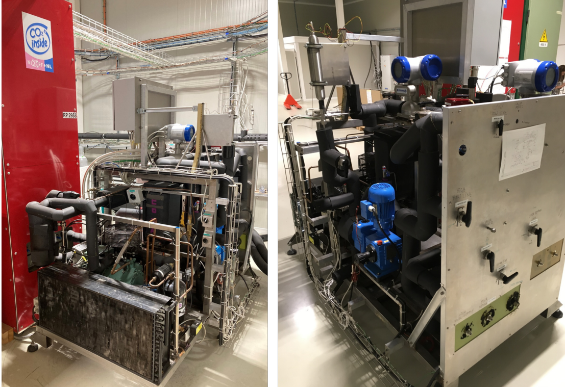
Figure 2.1 – Refrigeration unit CORA portrayed from different perspectives.
