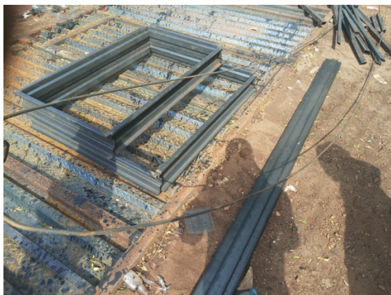
Welding – windows and gates
