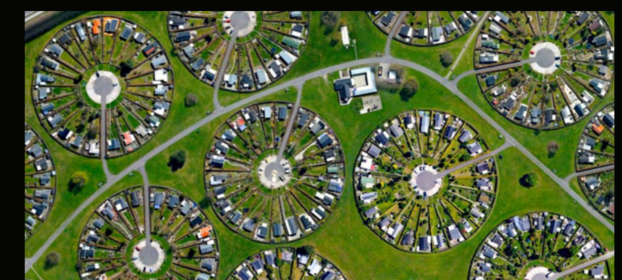
Brondby Garden City with a circular urban design (https://img.bfmtv)
